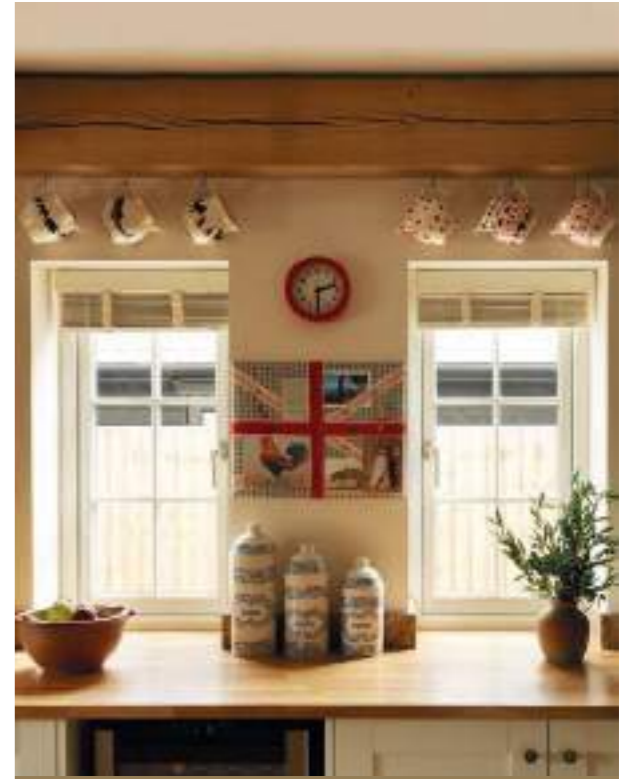
Flush casement windows painted in off white (RAL9010) and graphite black (RAL9011)
